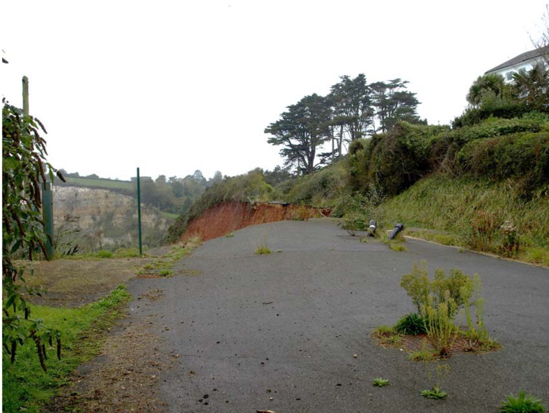
Figure 4e. CBU 3. White Haven landslide. View fom cliff top showing loss of c. 50m of Old Beer Road.
