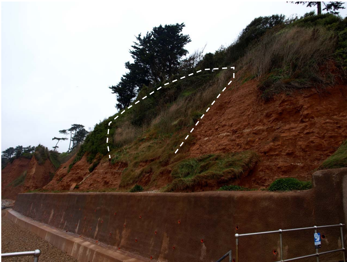
Figure 4h. CBU 6. Check House. Mudstone cliffs with two protection. Localised failures on the cliff produce fine grained sediment that may be delivered to the beach. Historical landslide embayment shown.
