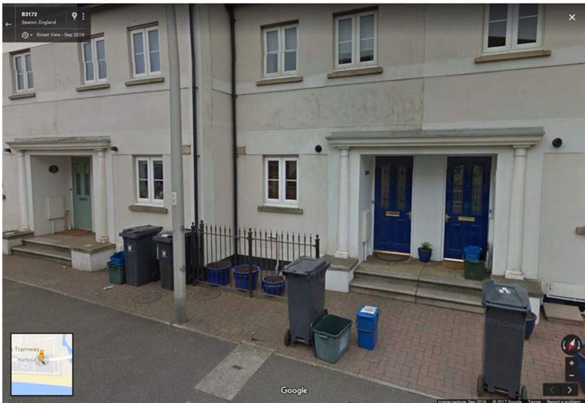
Figure 4: Residential properties along Harbour Road, Seaton (©2017 Google)
