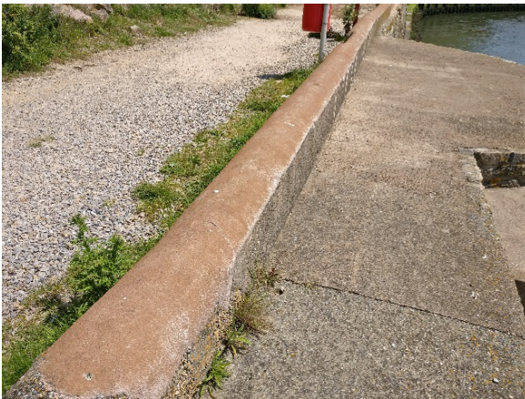
Patch repairs to the concrete flood wall
