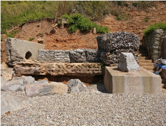
Rock at toe protection concrete slab and gabions
