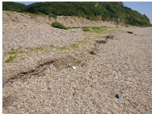
Cliffing was noted at the toe of the upper beach, exposing consolidated silt
