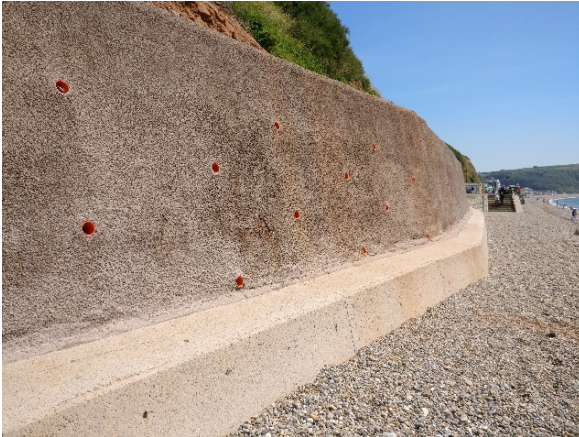
Sprayed concrete upper wall and reinforced concrete toe
