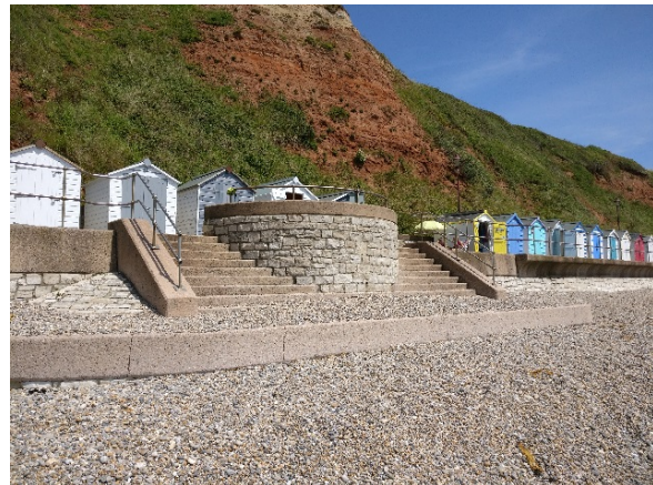
Typical stepped access in this frontage
