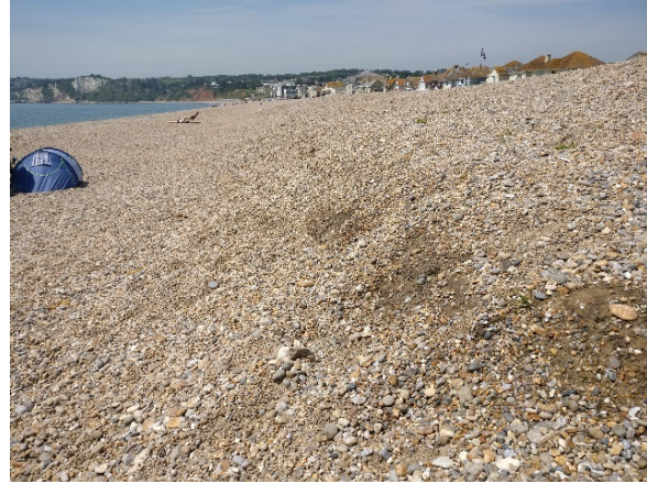
Beach steepens further east, exposing consolidated silt within the beach core (previous dredged material)
