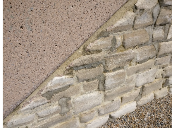
Patch repairs to grouting between stone blocks
