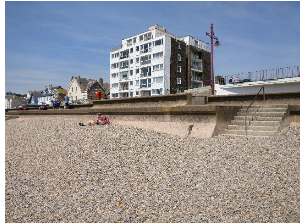
No signs of wall undermining, or slumping
