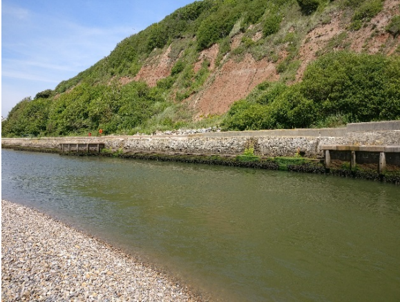
Stone block wall along the River Axe east bank
