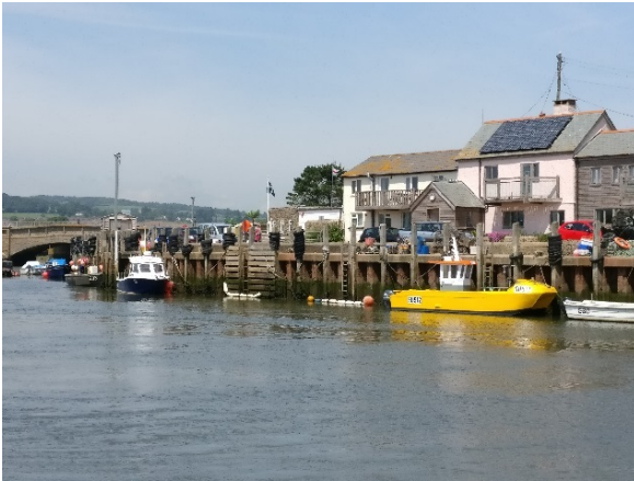
Steel sheet pile wall creates vertical defence
