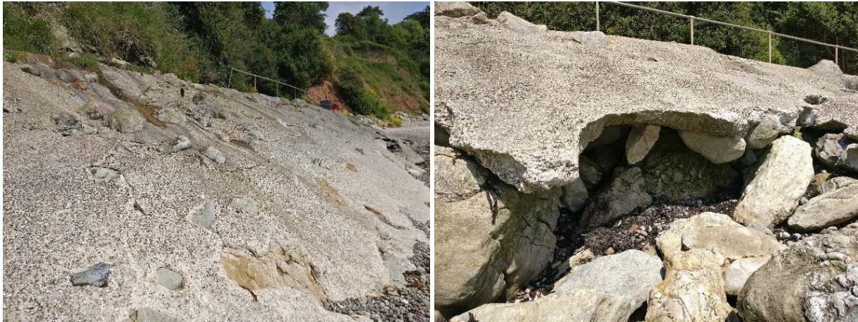
Figure 3-2 Seaton Hole concrete encased revetment
