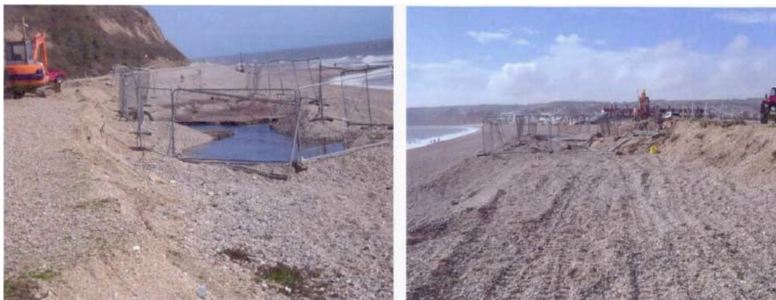
Figure 3-13 Trench for disposal of dredge material 2009/2010 Source: Author unknown 2, no date specified
