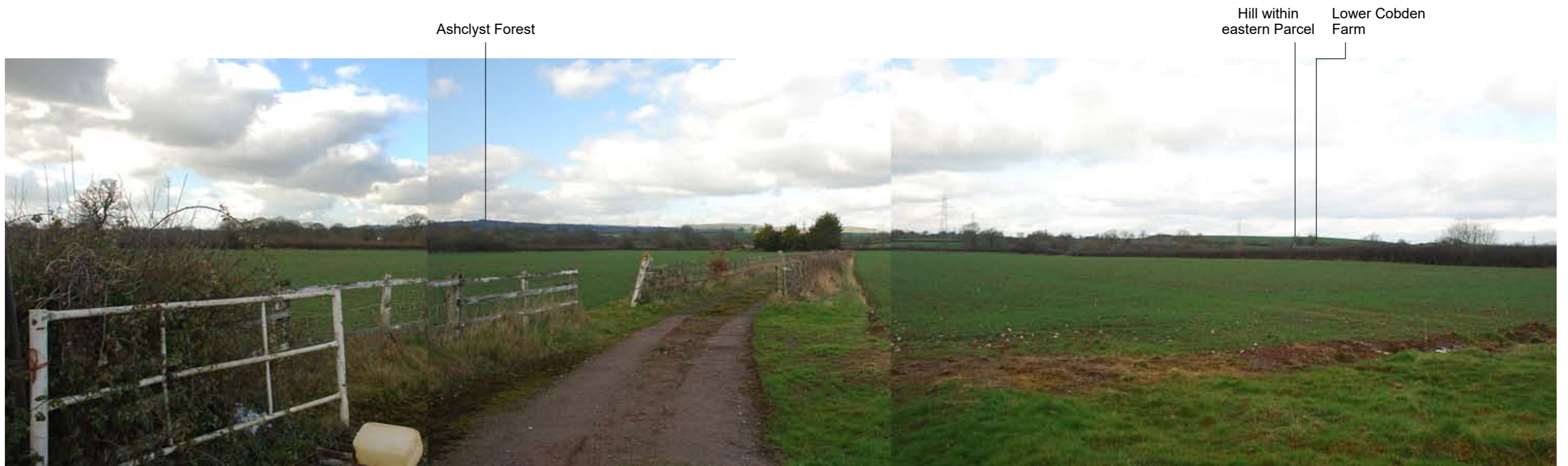
Photograph E4: Looking north from the southern boundary of the eastern parcel.
