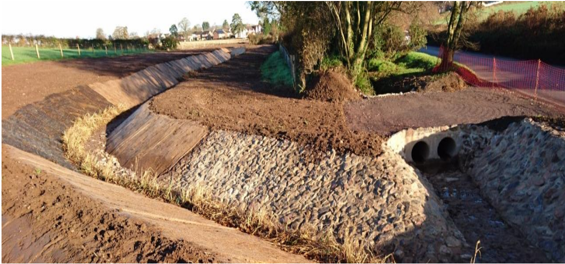
Flood alleviation works at Feniton
