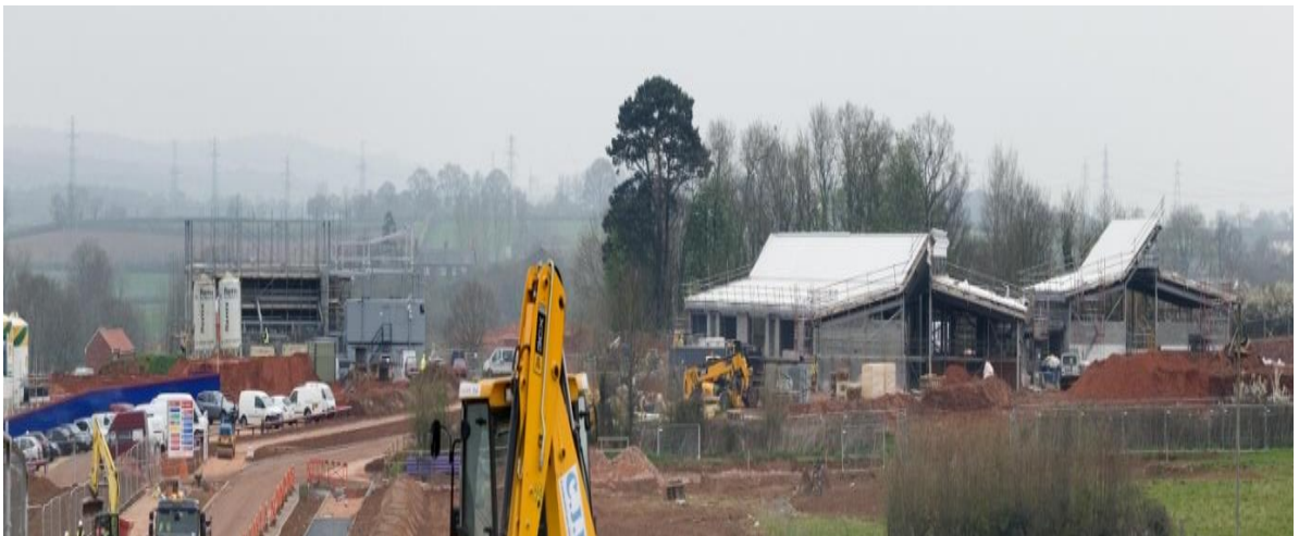
Construction at Cranbrook
