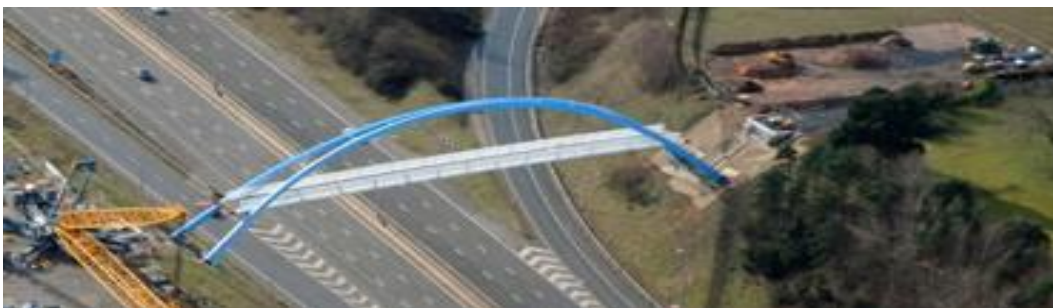
Redhays bridge spans the M5 providing a link for cyclists and pedestrians
