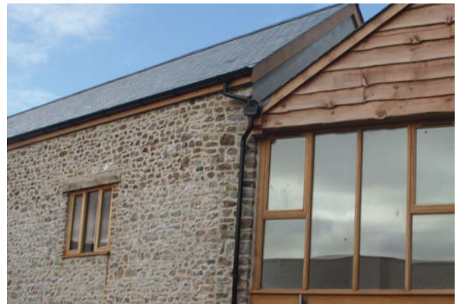
Successful conversions respect and reflect the building's original functions
