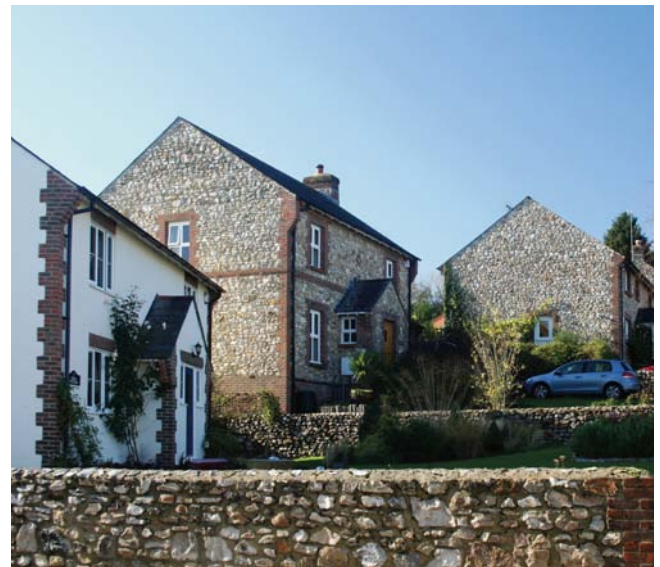
Modern houses, Smallridge reflecting local building styles and materials
