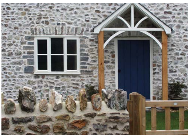
Restoration of an existing house in the Blackdown Hills
