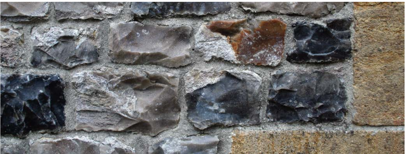
Flint with stone detailing, typical building materials in the Blackdown Hills, in this example laid in courses
