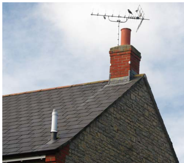
Characteristic gable end roof under modern slate
